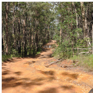
Existing unformed roads and drainage issues. Image: Lat27
